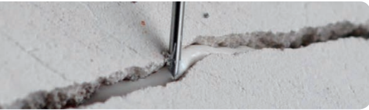
Filling of cracks
