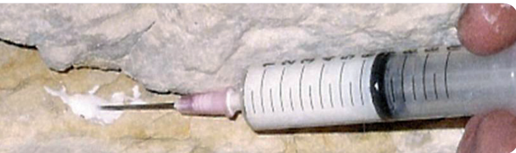
Backfilling with injection grout
